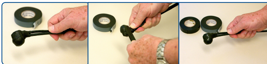
Figure 7. Taping a joint.
